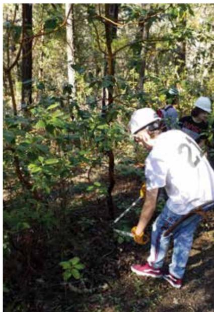
This student is determining the horizontal clearing line and removing limbs and small new growth that is in the tread zone. They also learned the vertical clearing limit for this trail in the campground.
