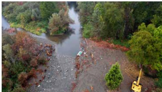
This shows the project site during construction. The dam has been removed and the irrigation headgate has been installed. The bare area on the right shows where gravel has been dug each year to build the pushup dam. This area will revegetate slowly over time. Photo: APWC.
